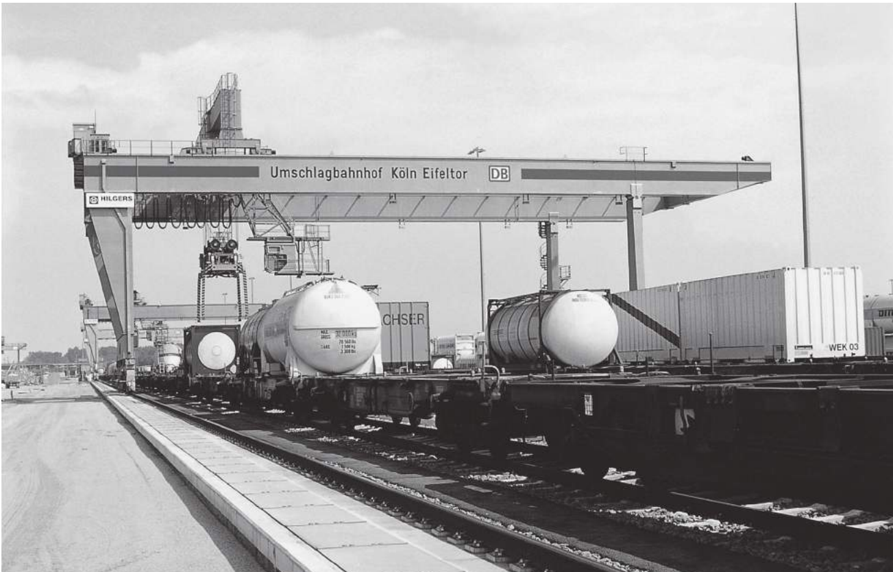
VAHLE-EID conductor trench for container terminal
